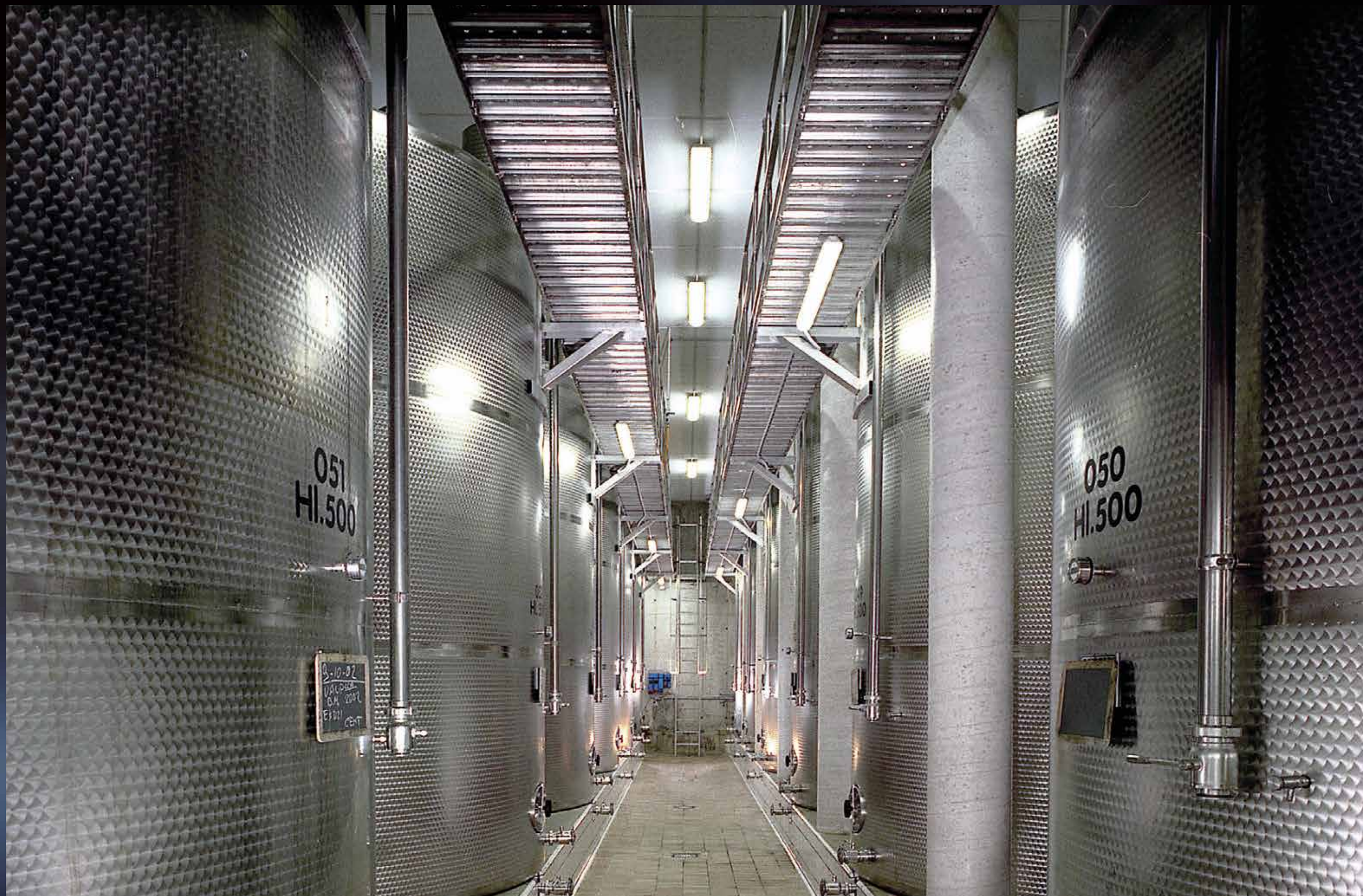
Wine cellar with 24 500 hl wine storage Megatanks
