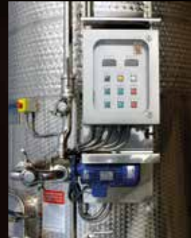
Electric board controlling the pump over pump and the punching down phases
