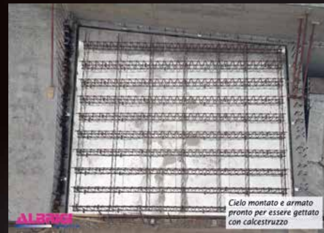
Installed and reinforced top ready for casting
