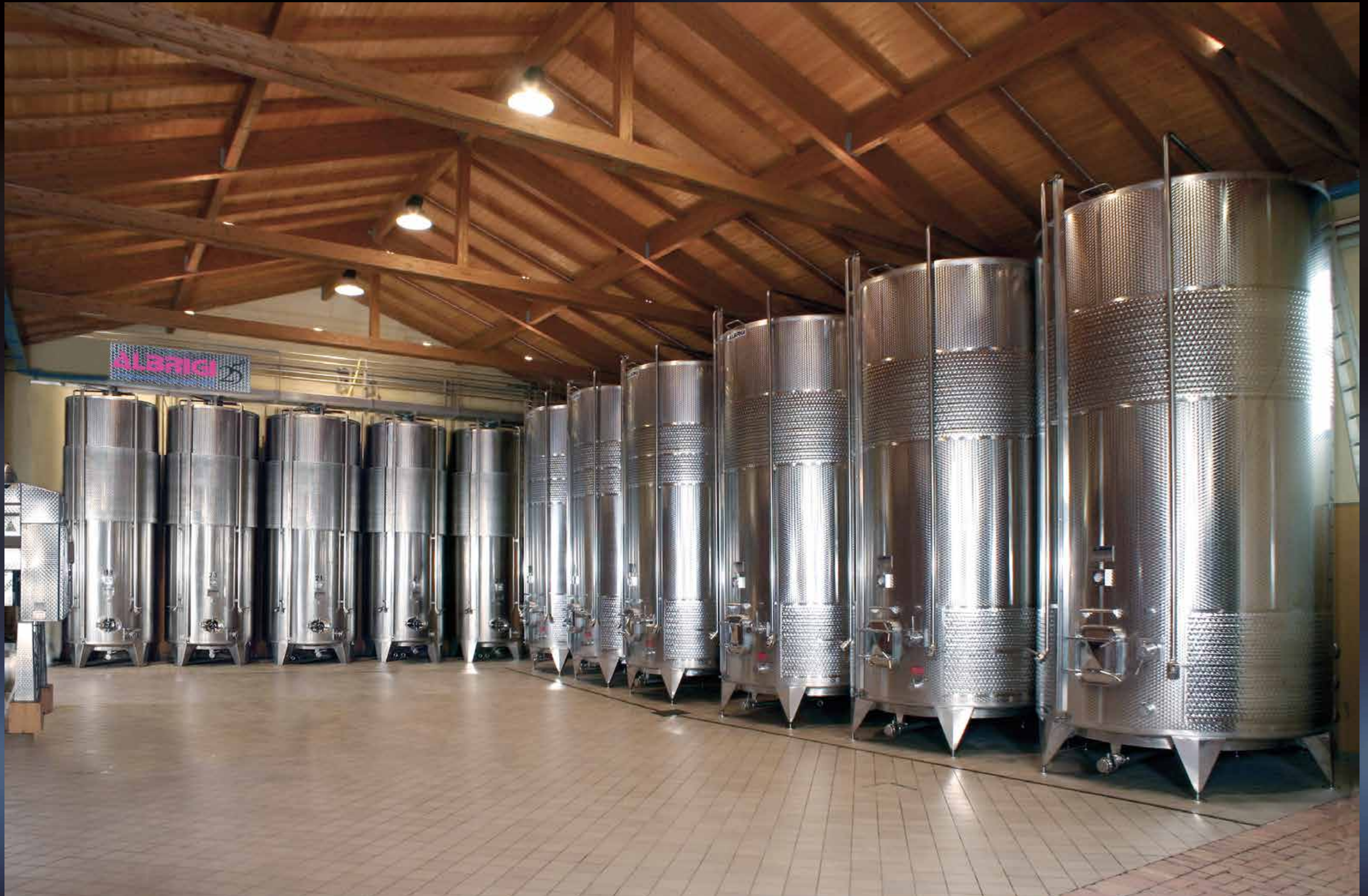
150 hl Termotank, temperature-controlled by Termostar and Isofix insulation 200 hl Termotank, temperature-controlled by Termostar Double, both equipped with Cleanfix washing plant
