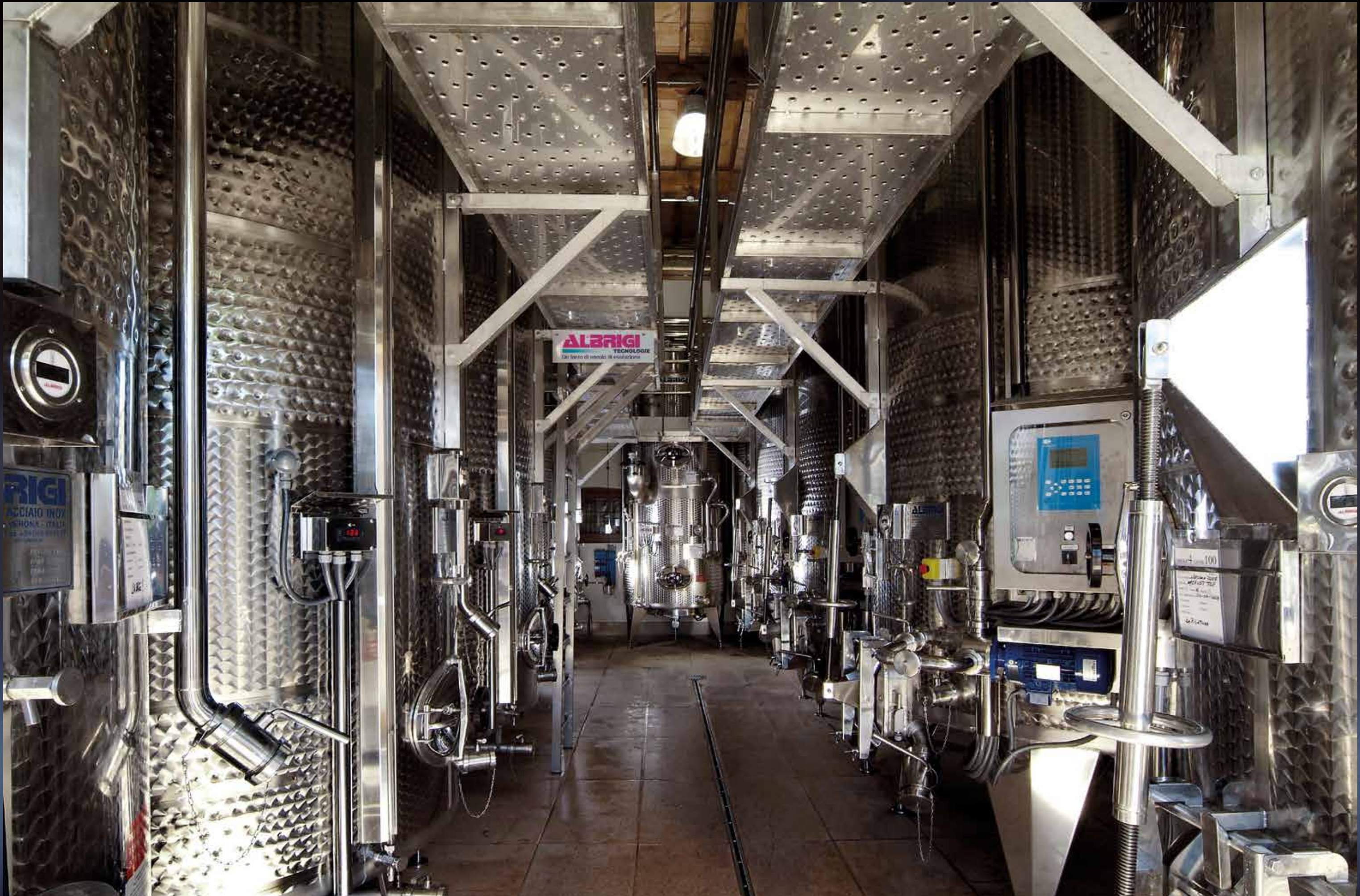
Meccanotank winemaking tanks with electric boards to control the fermentation processes
