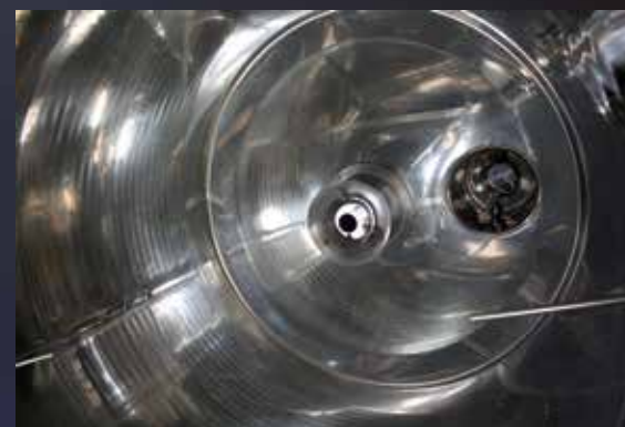
View of the upper compartment from below
