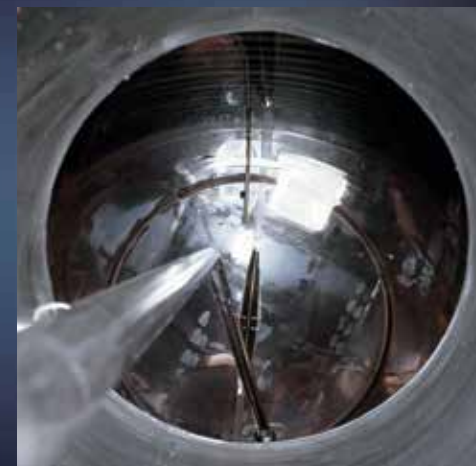
View of the lower compartment from above
