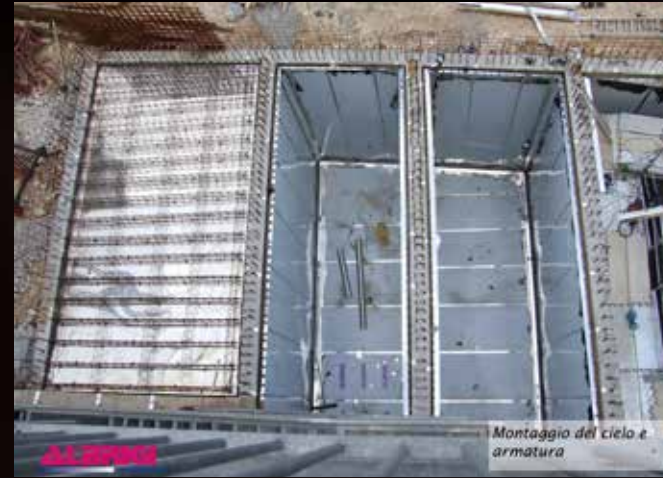
Installed and reinforced top ready for casting
