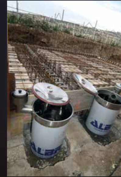
Installed and reinforced top ready for casting
