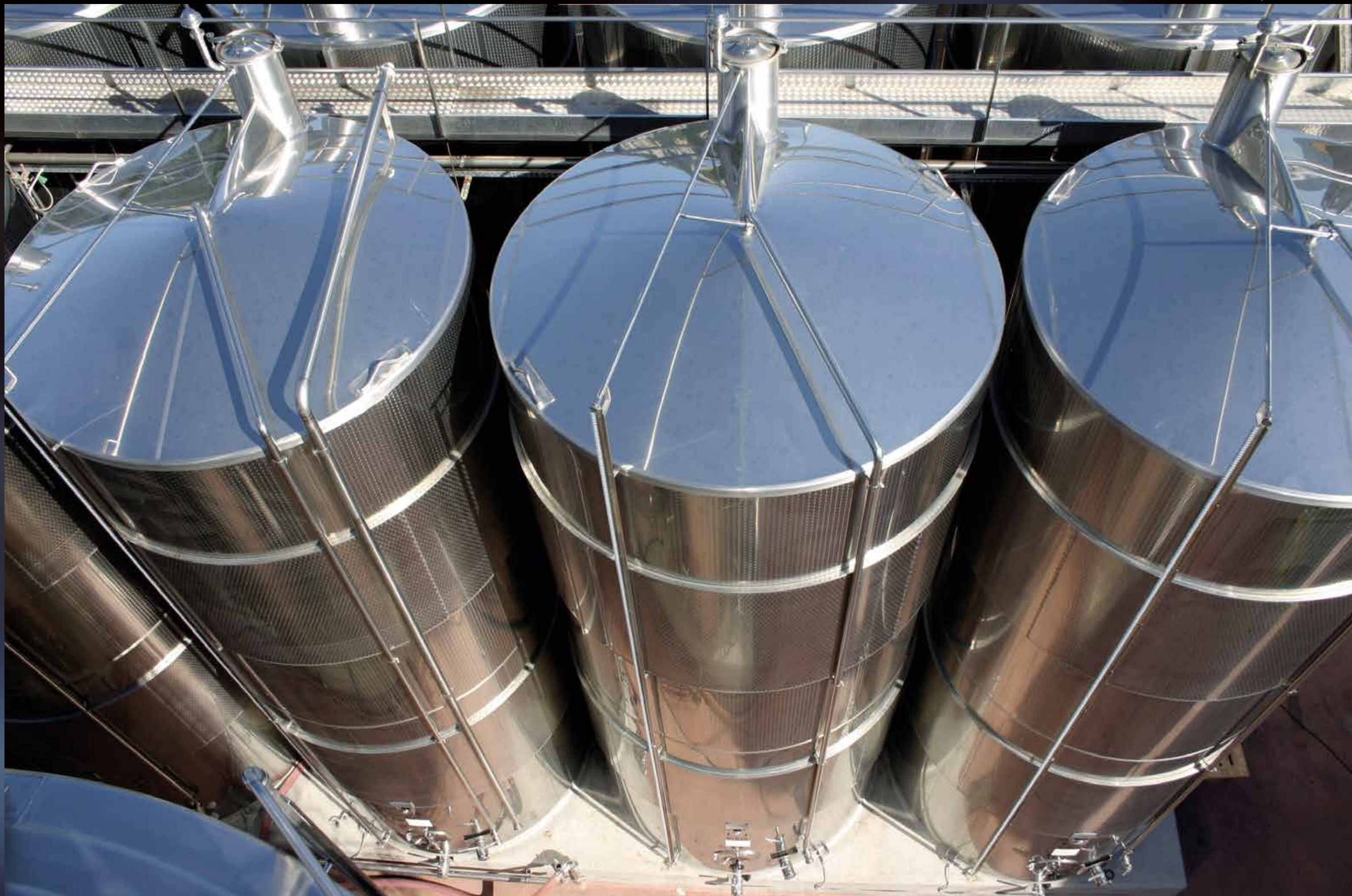
600 hl Megatank, temperature controlled by Termostar Double, fitted with Isoplus Insulation and Cleanfix washing plant
