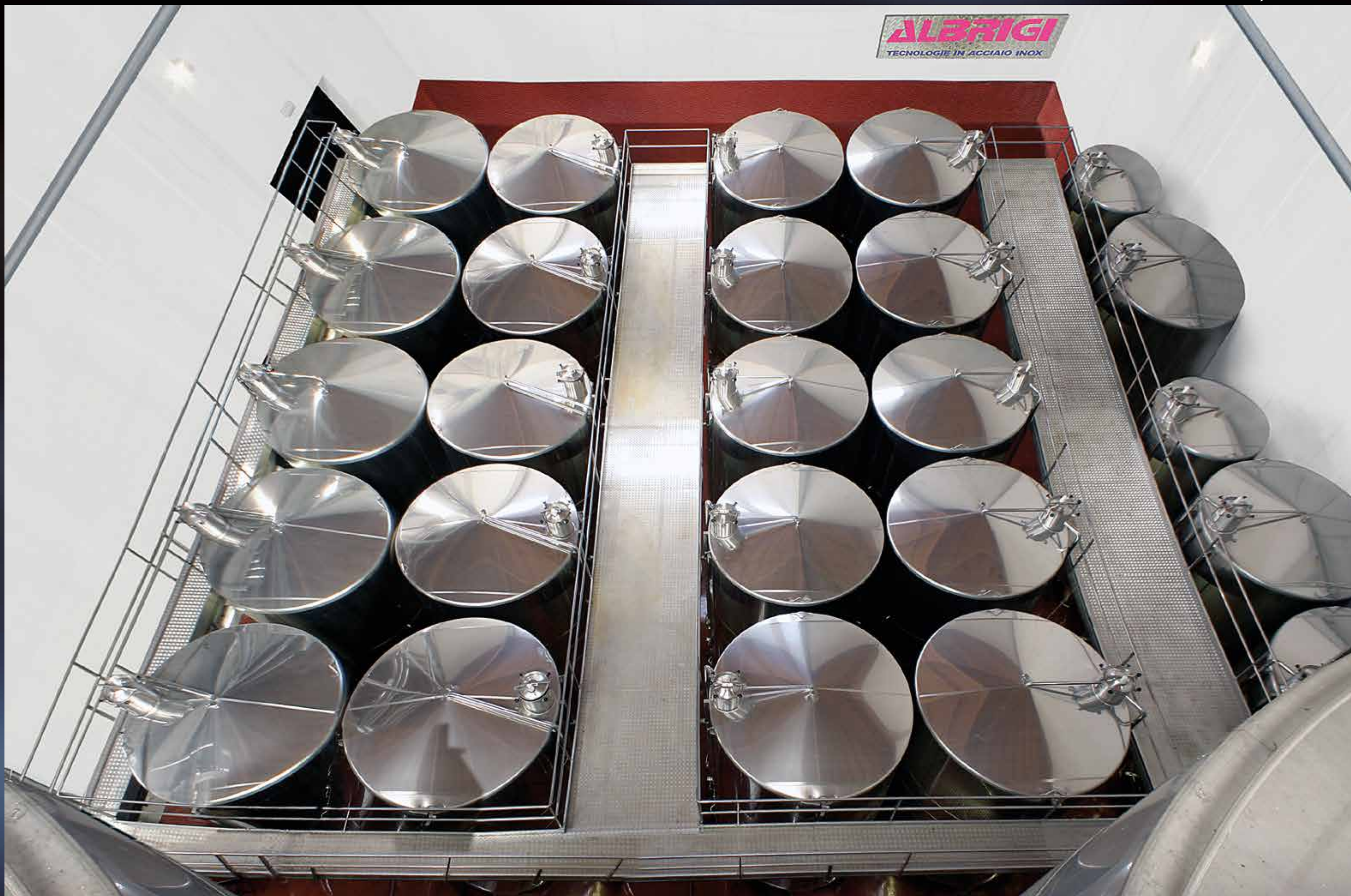
Storage wine cellar with 300 hl Vinotank with Cleanfix washing plant
