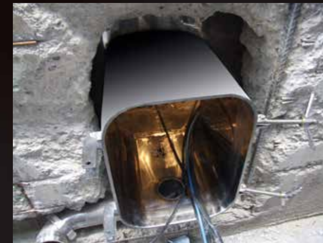
Installed and reinforced top ready for casting
